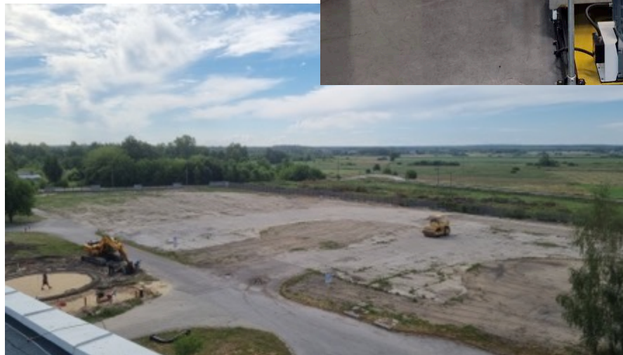
Land cleared for solar park Kozienice, Poland
